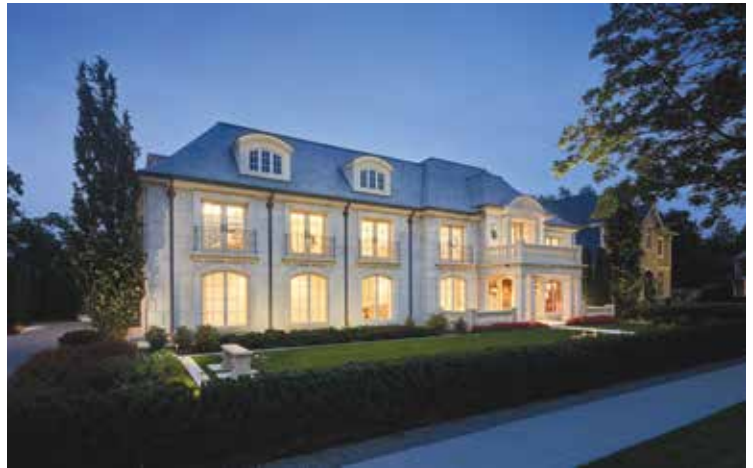
DesRosiers Architects | 3RD
